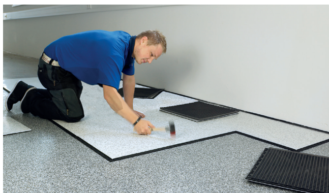
Tip: Laying with soft-head hammer
